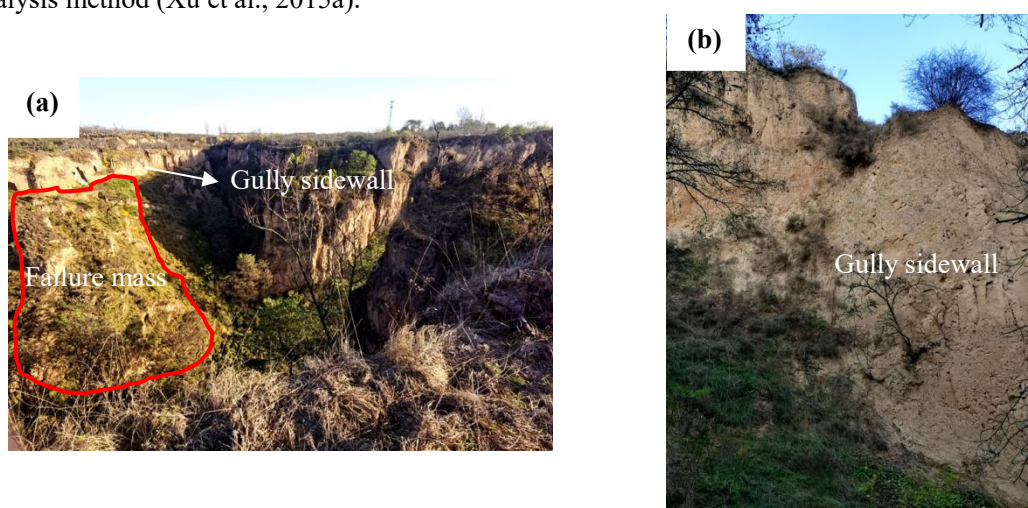
Figure 1 Photographs showing the representative loess gully sidewall on the Loess Plateau of China. (a) Gravity erosion on the gully sidewall, and (b) a typical gully sidewall with a slope gradient of more than 70^\circ .
